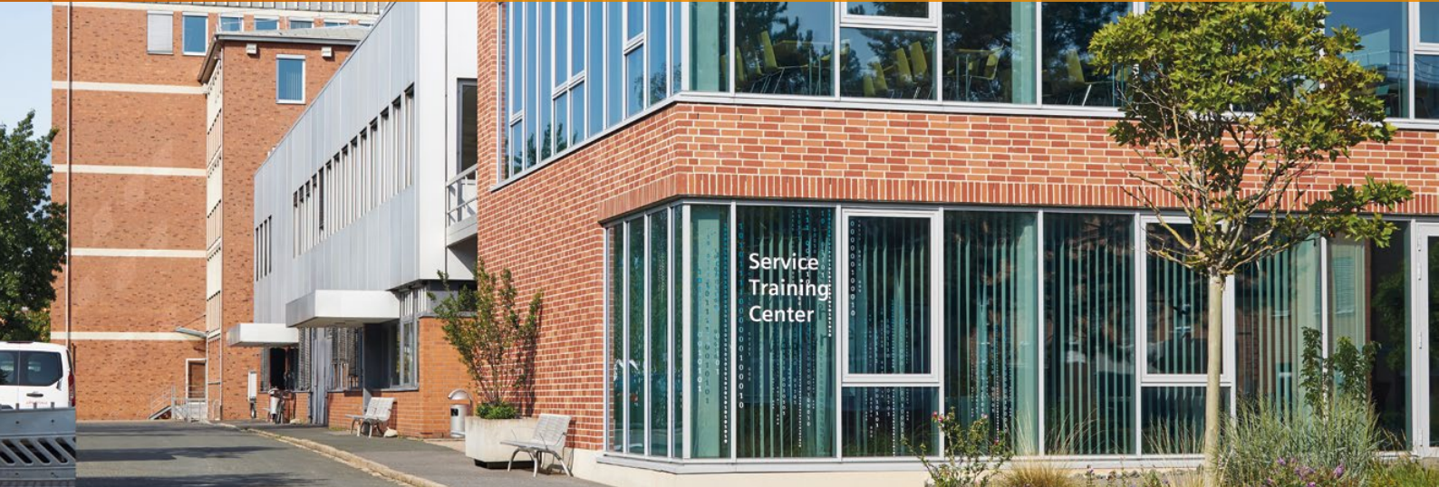
Siemens Technopark Nürnberg (Source: Siemens Real Estate)
