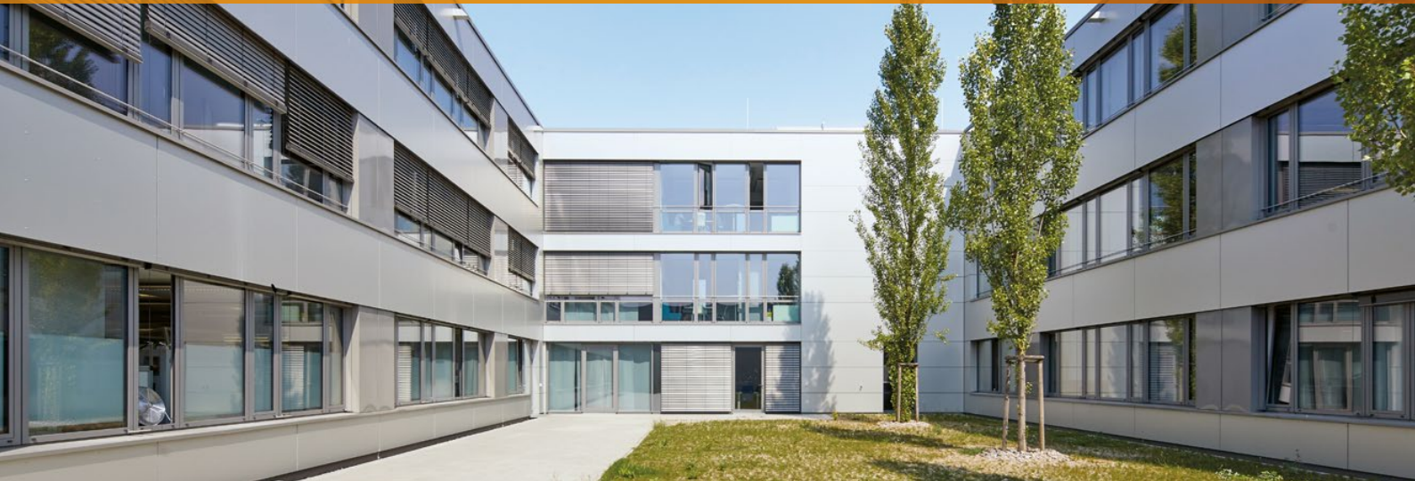
Siemens Technopark Erlangen (Source: Siemens Real Estate)
