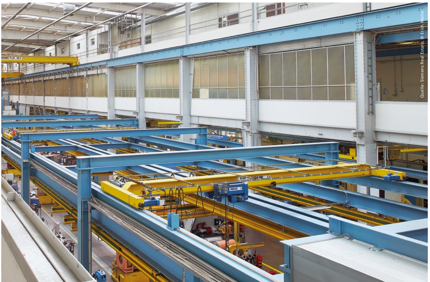
Innenansicht einer Produktionsimmobilie in Nürnberg Interior shot of a light manufacturing property in Nuremberg
